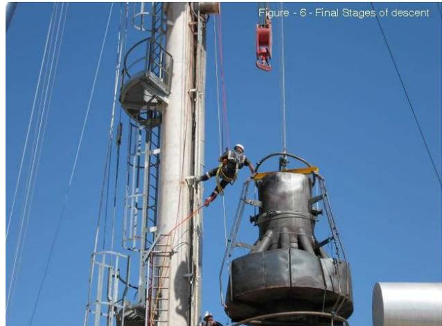
The installation of the replacement flare tip was completed in reverse order. Figure 7 (photographs) depict the final installation of the new arrangement.
