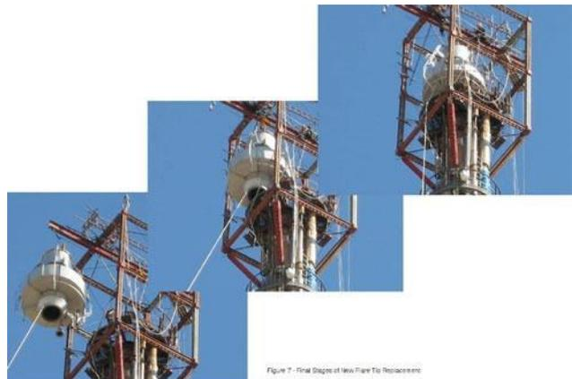
On completion of the works the lifting davit was lowered to grade level, labelled and packed in a site container for future deployment.
