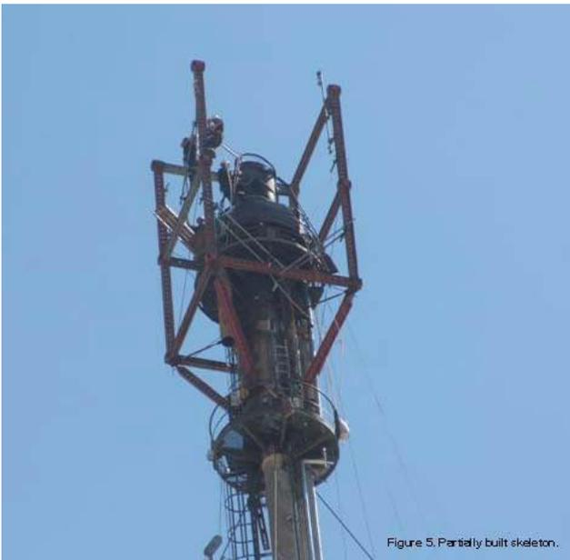
Following erection of the lifting davit skeleton, the runway beam was installed above the flare unit. The completed arrangement was inspected and tested prior to use. A number of further checks were also completed.
